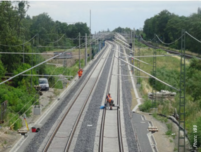
Workers completing the Dresdner Bahn section between Berlin-Südkreuz and Blankenfelde
