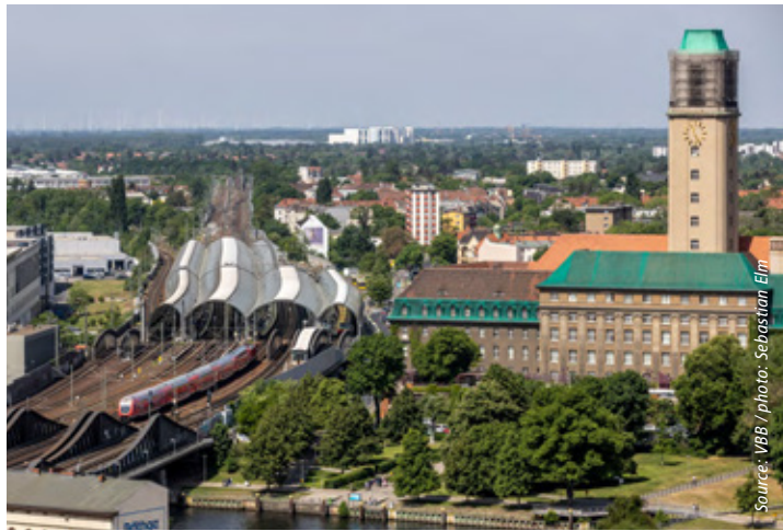
Berlin-Spandau station is getting two new platform edges
